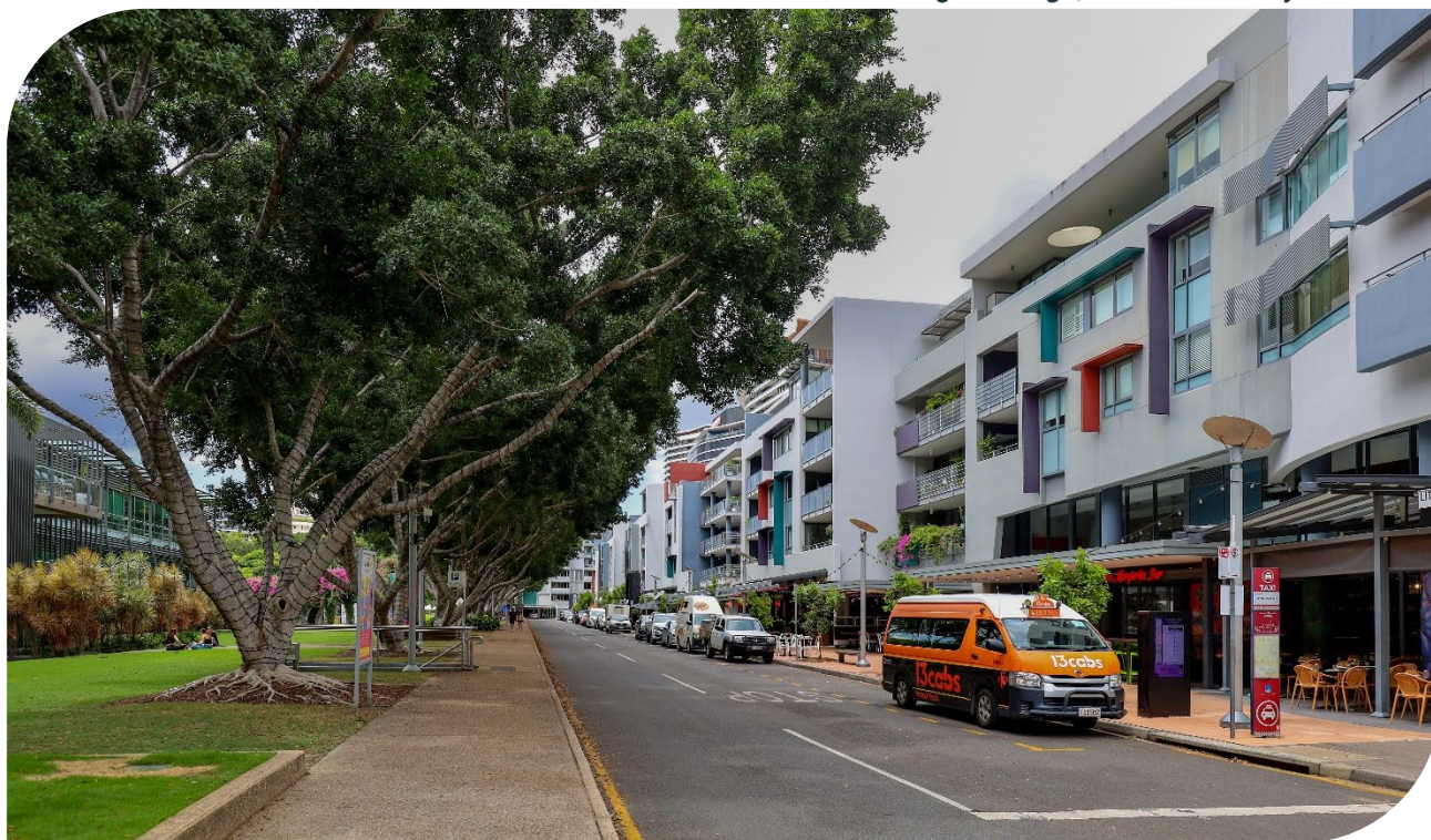
Figure 29 Example of mixed-use with active frontage, and wide landscaped active transport corridor adjoining road frontage, Southbank
