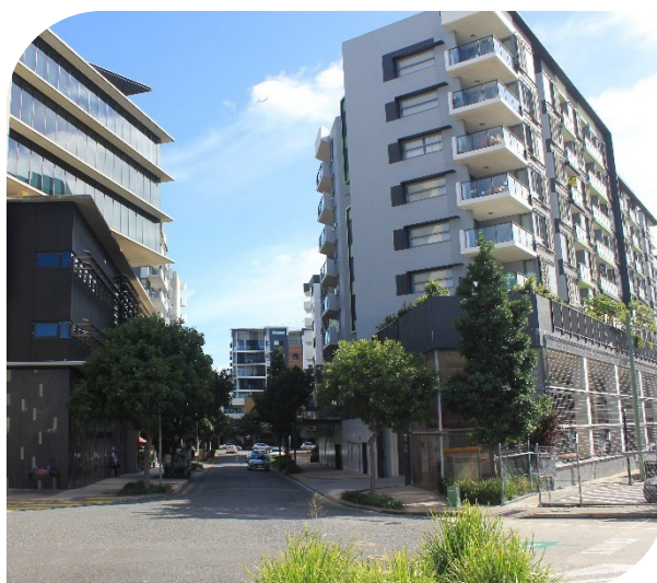
Figure 15 Example of ground floor carparking screened from active street frontage, Nundah
